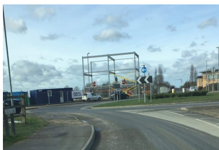
Shaping up nicely: a picture of our build shared on Facebook this week.
